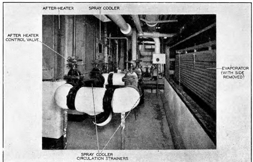
FIG. 3.—VENTILATING PLANT.
