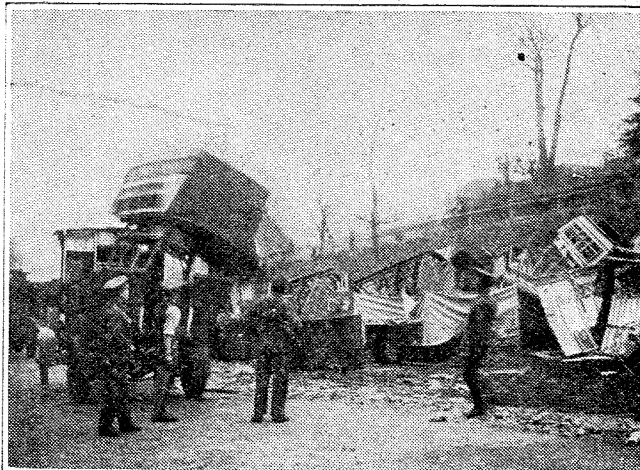
How a London motor-'bus is adapted for active service. The top is removed bodily. A little sawing, some strong rope, and a hefty pull, and the "General" is quite ready to do its bit for the country.
