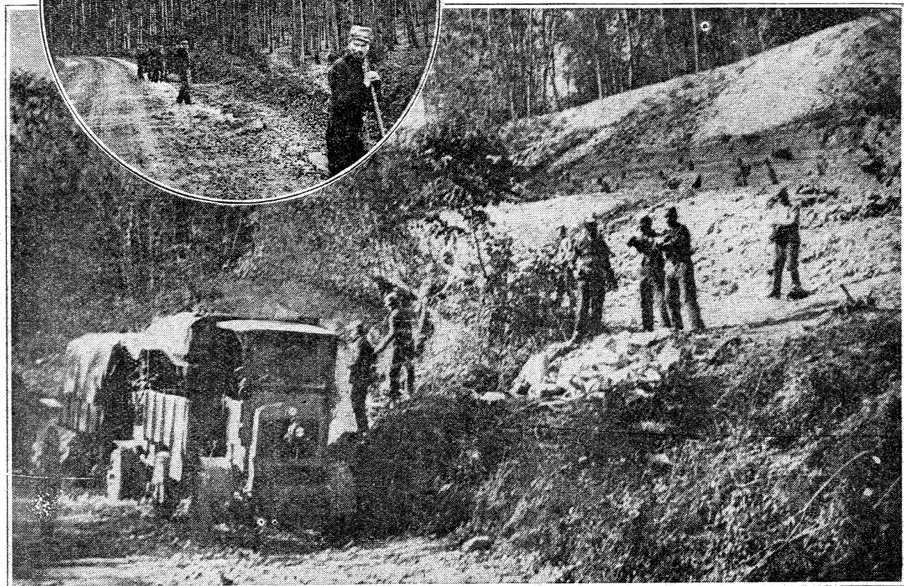
Digging a three-decker entrenchment, typical of many in the Argonne, where undulating ground lends itself particularly to this form of trench construction, which is considered to be impregnable. Inset: French engineers at work by the wayside in the beautiful forest.
