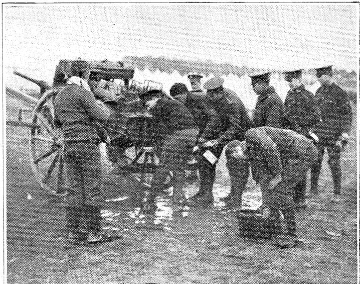
Precautions against enteric. The latest innovation of our perfectly equipped Army. A travelling filter to ensure purity of drinking-water.
