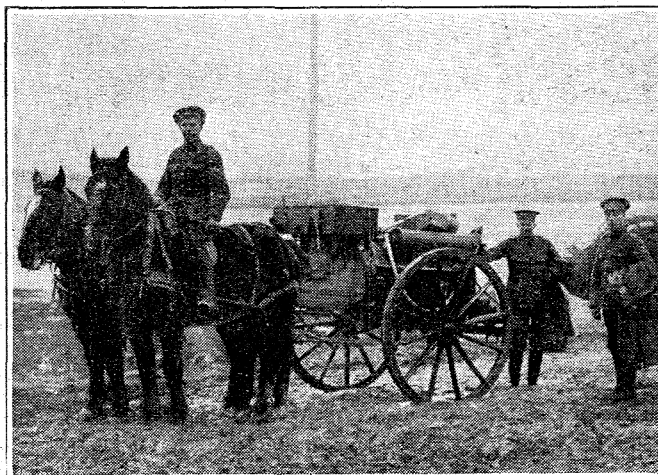
One of the special filter water-carts which supplies pure unadulterated drinking water to the army if wanted at any time.
