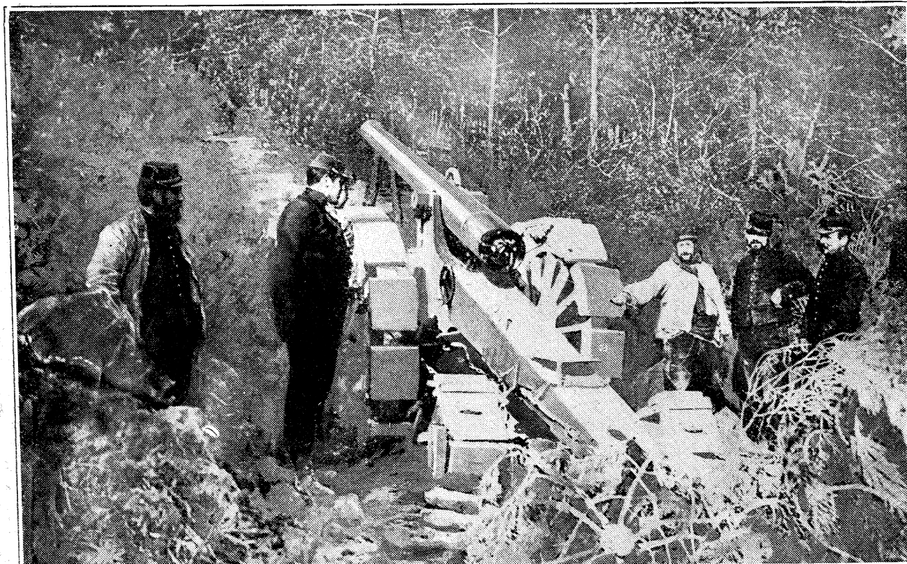
French gunners about to fire one of our allies' large cannons in the Forest of Argonne. Like the great German siege-mortars, this weapon is fitted with wheel-pads to assist in its transport, the eternal problem with heavy machines.
