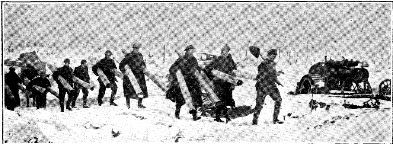
These warmly-clad Tommies of a working-party are not carrying Brobdingnagian cigarettes, but stove-pipes for use in huts, shelters, and workshops behind the lines, where fires are much needed in such wintry weather. They are just passing one of their big guns.
