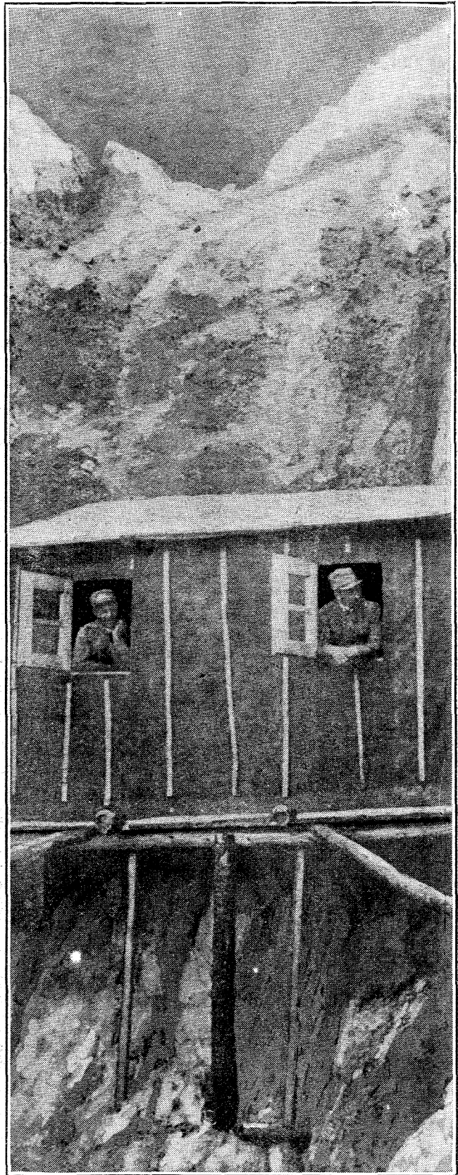
Remarkable, too, is the feat of engineering shown at the terminus of the long ladder, where this outlook hut is fixed in a cleft in the very face of the mountain. Though their quarters must be somewhat cramped, the Italian soldiers evidently maintain a smiling front at their lofty and lonely post.
